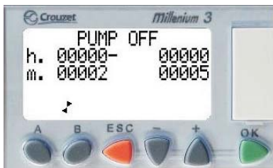
Minimal Level Fault Signal
