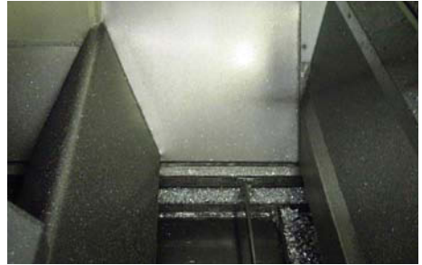
Figure 24 Large area openings in the chip conveyor
